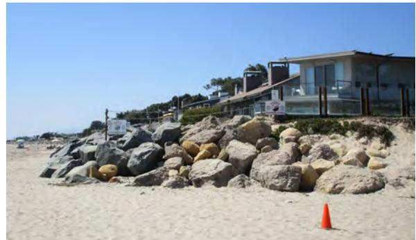
*Rock revetments are considered a “hard” coastal protection structure that fix the shoreline in place and buffer coastal resources from severe storm events.*
